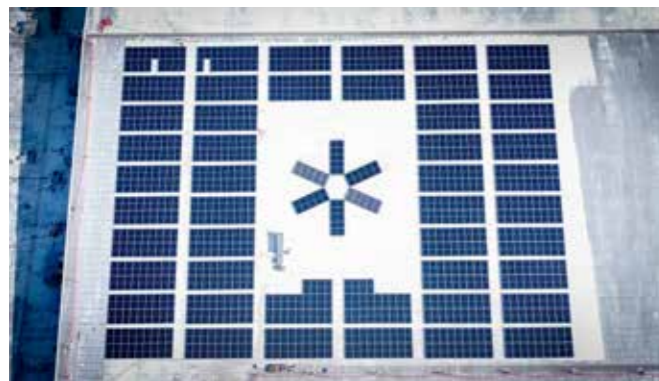
ROOF-SOLAR TPO / 499,22 kWc Costa Rica
