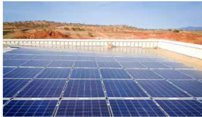
ROOF-SOLAR BITUME / 151,7 kWc Maroc
