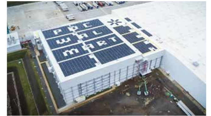
ROOF-SOLAR TPO / 208,8 kWc Costa Rica
