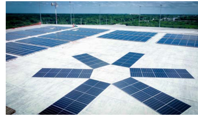
ROOF SOLAR TPO / 500 kWc Costa Rica
