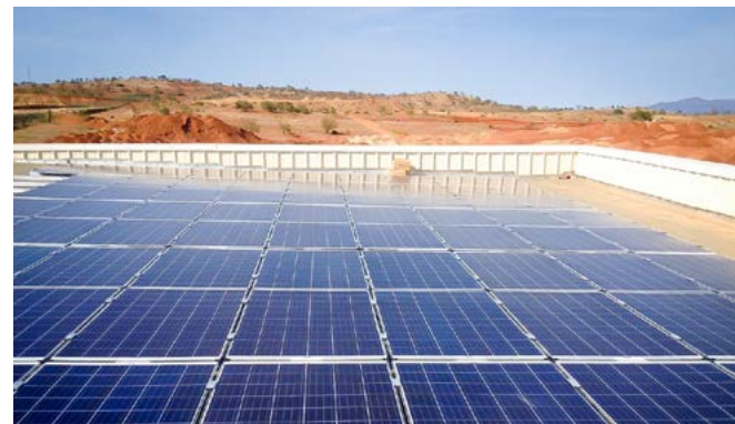
ROOF SOLAR BITUMEN /151.7 kWc Morocco
